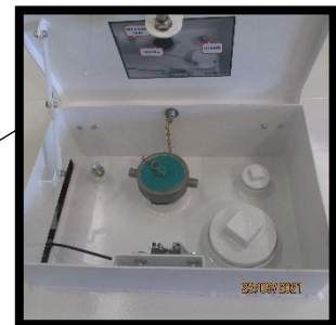
Refilling and Dip lockable cabinet including 3" Dip and Fill Cap with lanyard chain, Spare 2" port and Roll over vent
