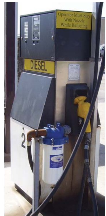
VF-61 connected to a diesel fuel dispenser
